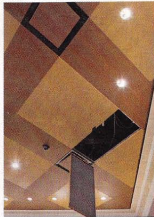
Metal panels swing open for easy plenum accessibility at Lumière Place.
